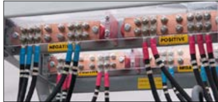
24 V Cable harnesses and bus bar illustrated
