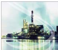
Building & Industrial Plants
